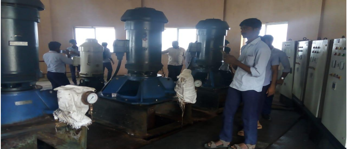
Industrial Visit – 16.02.2019 at the KL Rao Water Treatment Plant Civil III year II semester students along with Faculty
